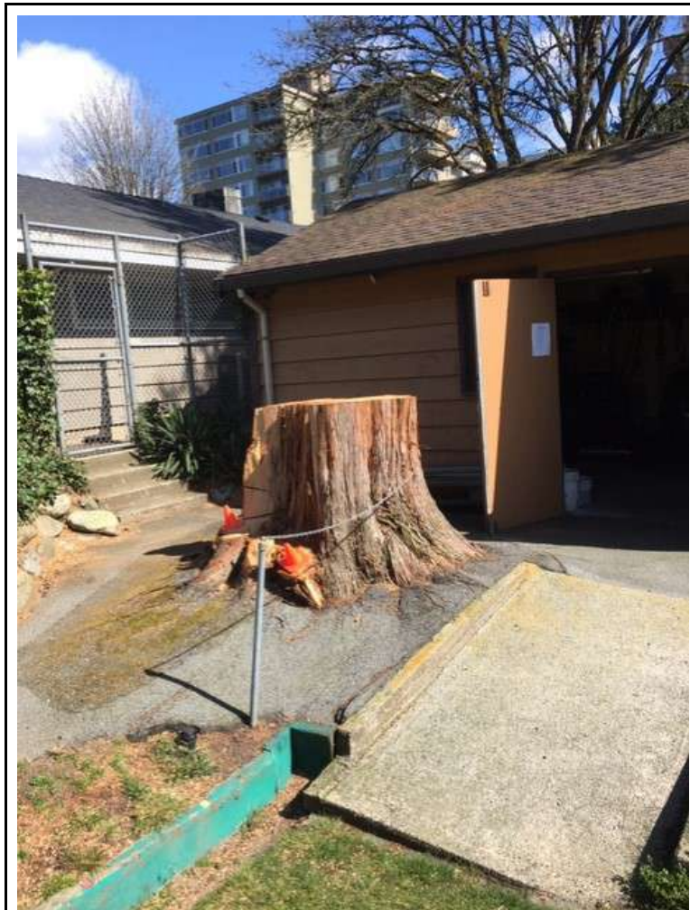
Repairs have been made from the March windstorm
